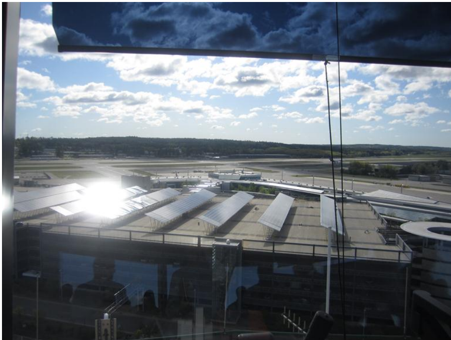
Figure 22. Glare viewed from Air Traffic Control Tower at Manchester/Boston Regional Airport (~8:17 AM EDT, 5/10/12). Note that tarp has been placed over some of the modules.
